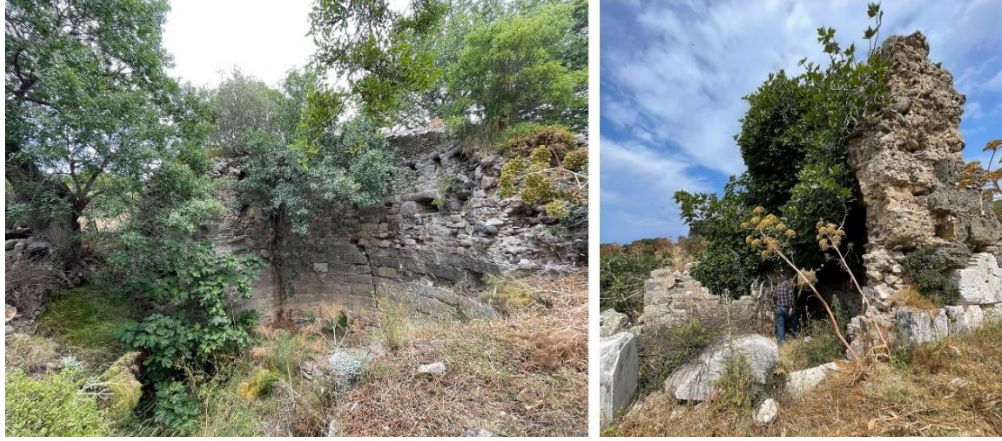
Figure 26: Bath and Church structures damaged by fig trees and weeds
