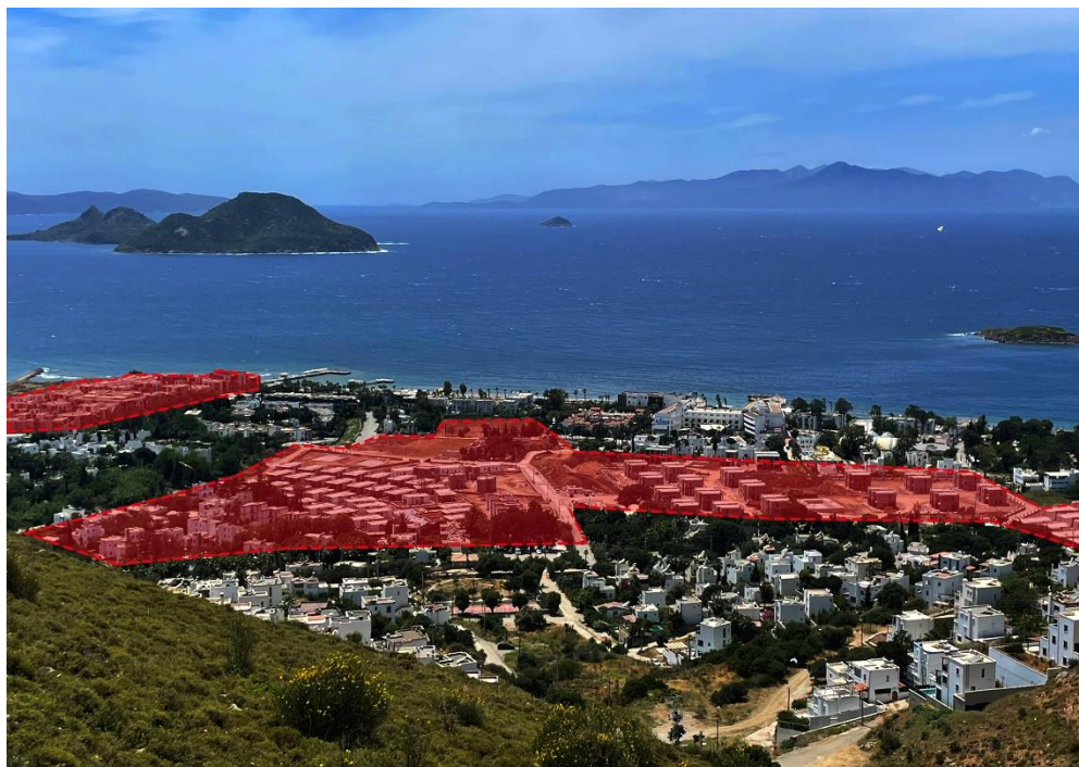
Figure 32: A photo from Kadikalesi (Peksimet) which shows dense construction activities around so-called old Myndos
