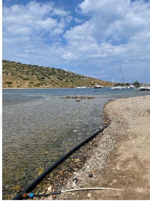
Figure 22: Laid pipelines as a marginal solution to lack of infrastructure
