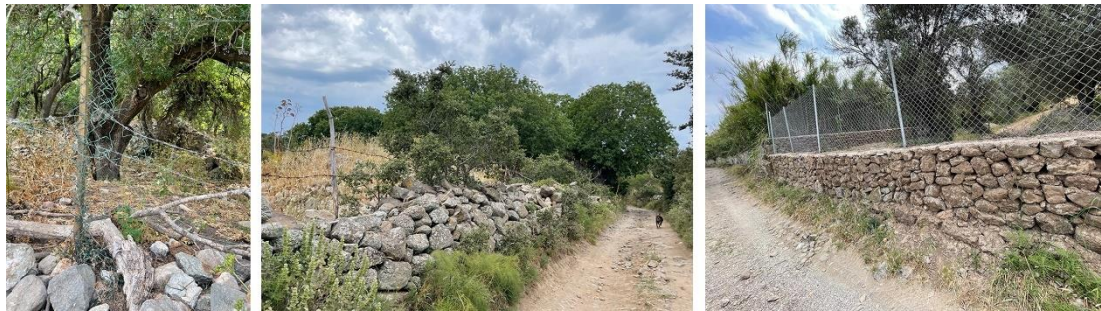
Figure 25: Wire fences as protection measure in Myndos
