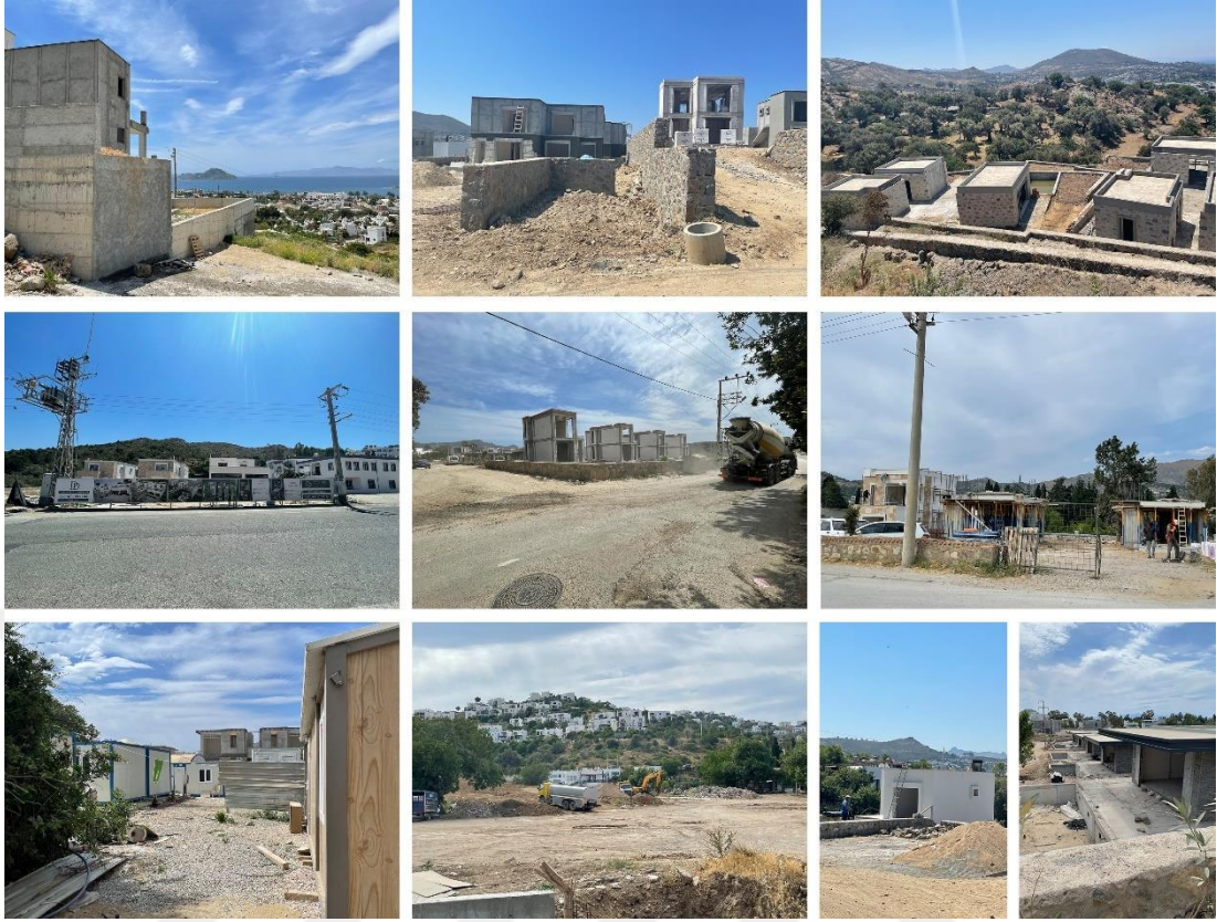
Figure 33: The photos of dense construction activities from Peksimet
