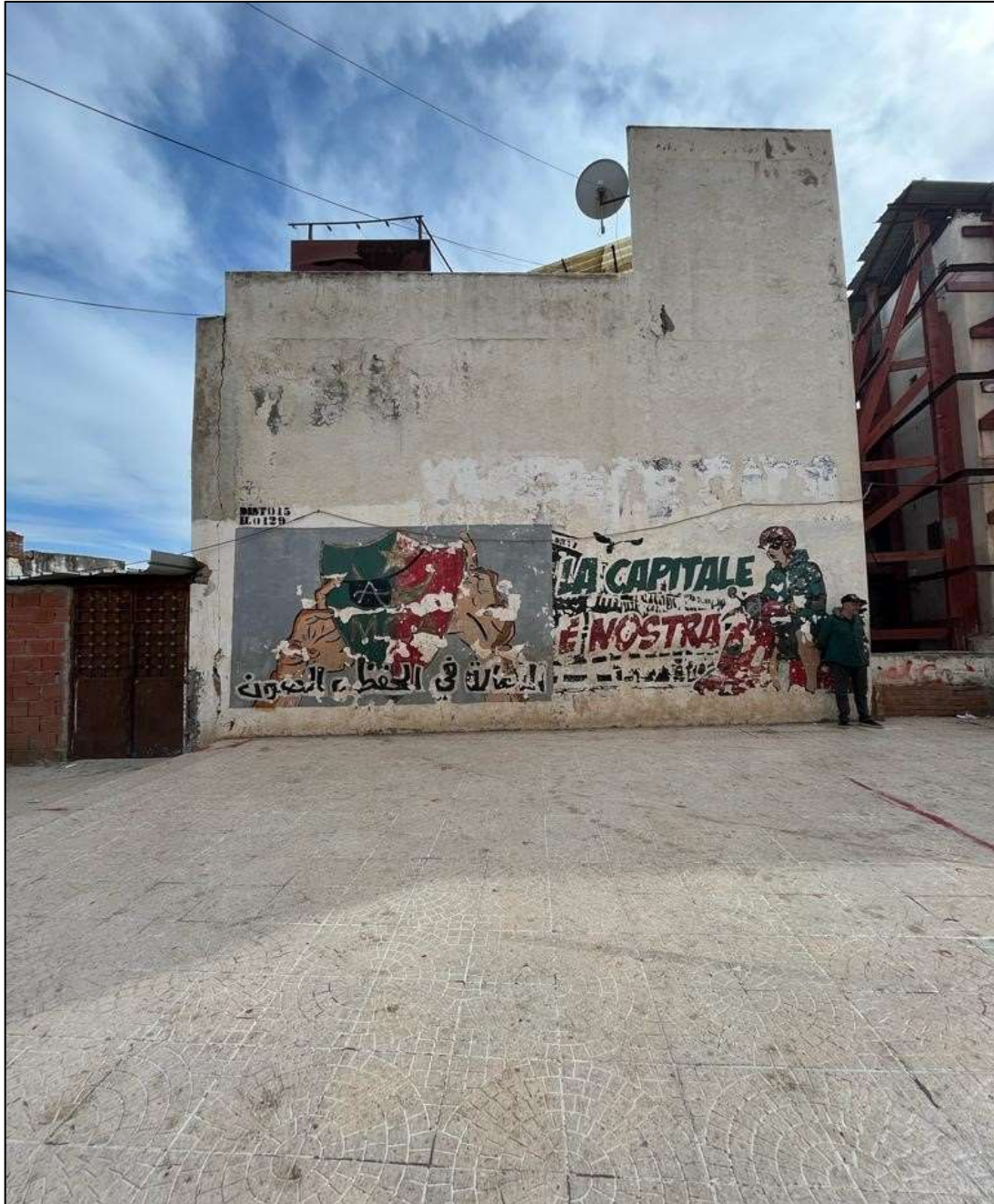
Figure 4.29: Picture Showing the Void in Plot Number 4.
