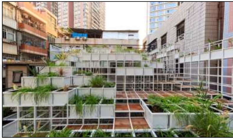
Figure 3.9: View on the Roof Transformed as Public Space (Shuang, 2018).
