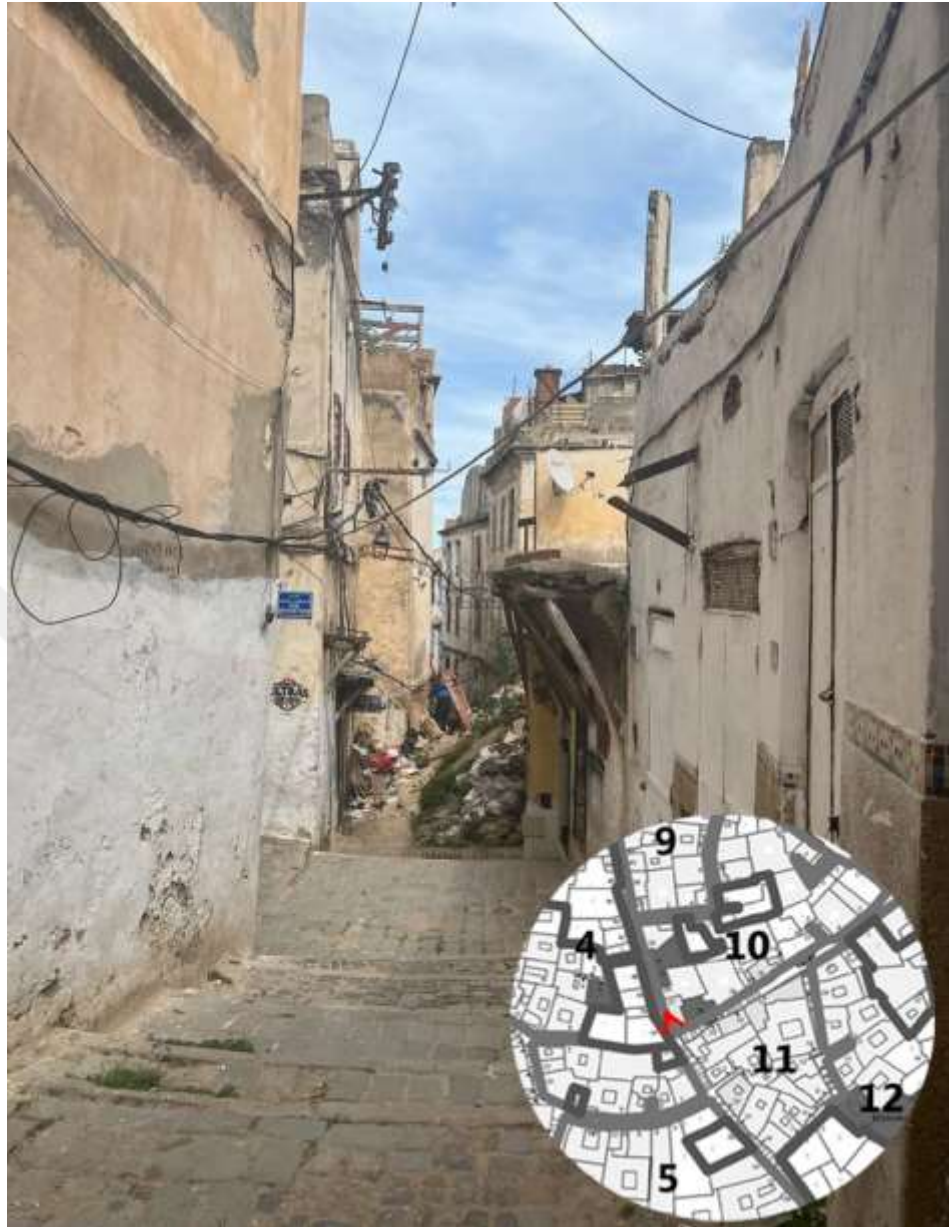
Figure 4.26 Collapsed Building-View From Street R.Riah.
