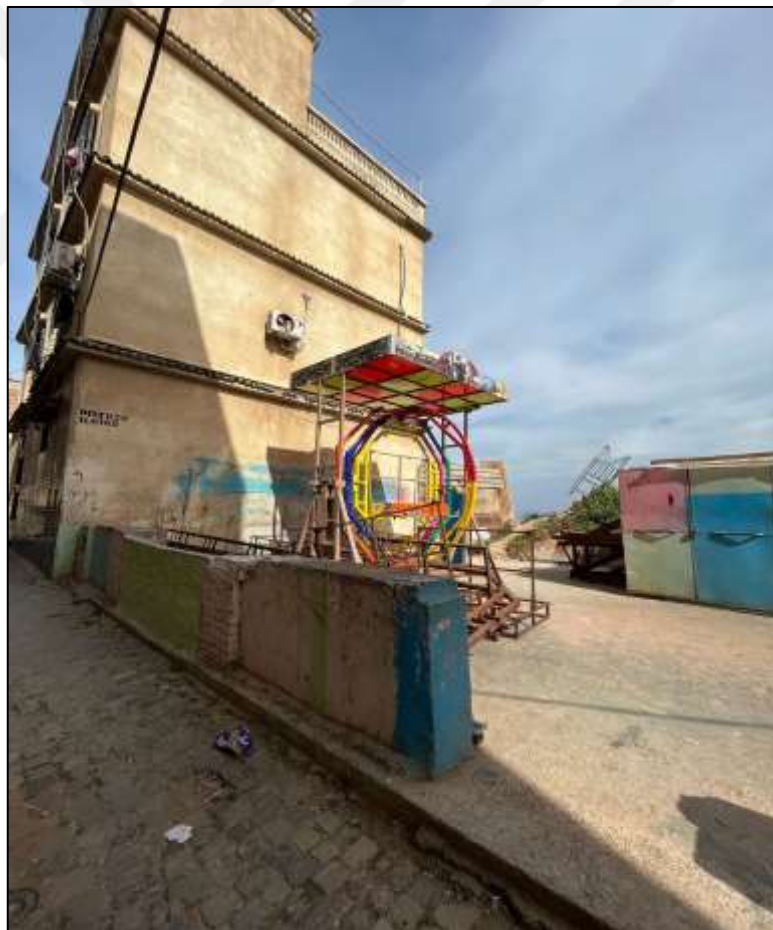
Figure 4.37: View of the Open Workshop.
