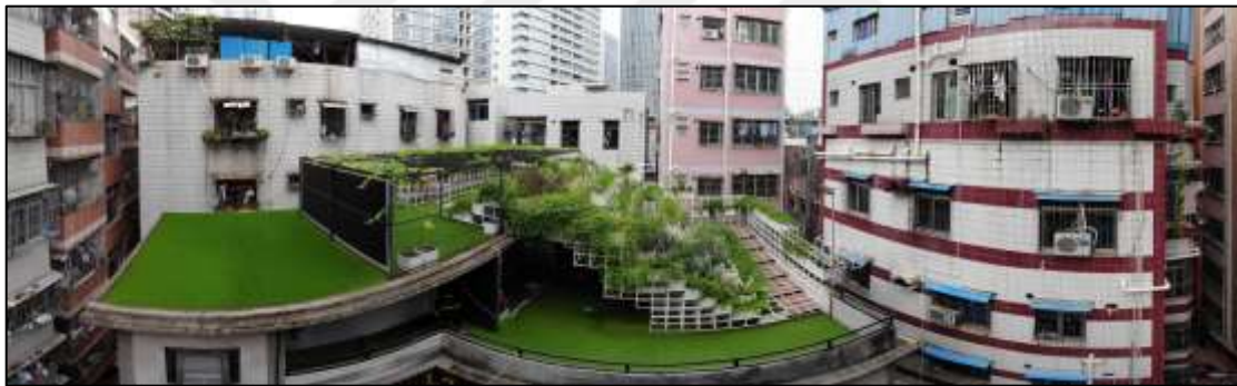
Figure 3.12: View on the Roof and the Surrounding Building (Shuang, 2018).
