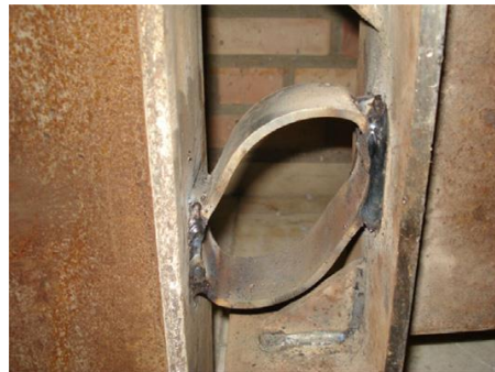
Typical deformed shape of bare steel pipe specimen
