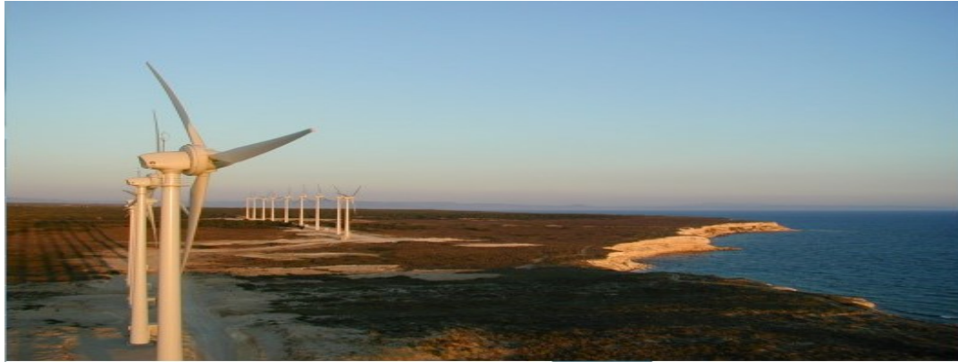
Figure 4.1 Established Onshore Wind Farm 3
