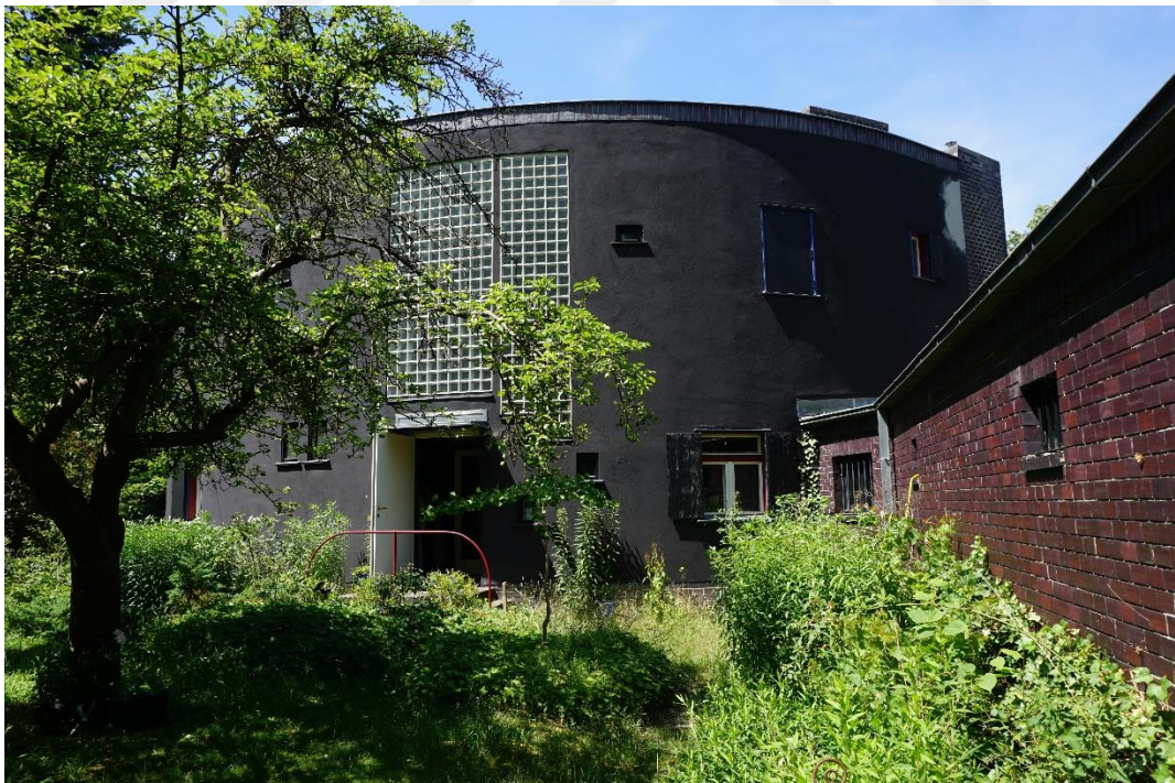
Figure 10: Front facade of Dahlewitz. Source: The photo was taken by Yıldız Kılınçer, June, 2019.
