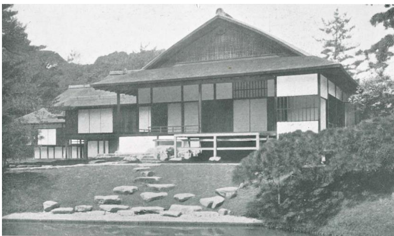
Figure 20: The moon-terrace and the main gable of the building stand out in all its beauty. Source: Houses and People of Japan, 1938, p. 291.
