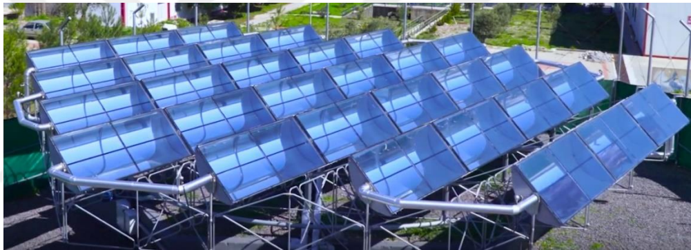
Figure 2.12 Parabolic trough collector plant in Izmir Teknopark (Lucida Solar, n.d.)
