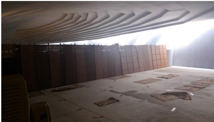
Figure 4.4. The screens added to the women's section
