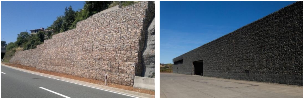
Figure 3.29. Former uses of Gabion Wall as retaining (left); Dominus Winery – Herzog & de Meuron (right)
