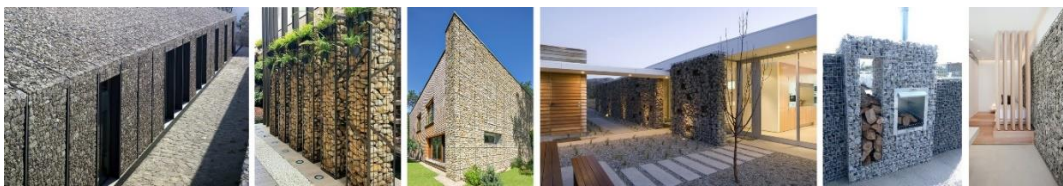
Figure 3.30. Prevalent use of Gabion Walls
