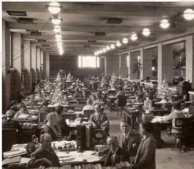
Figure 2.1. A typical Taylorist Office (Lovell, 2017)
