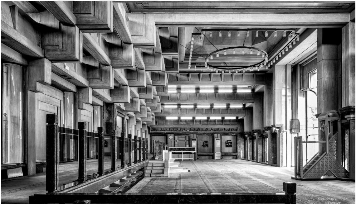
Figure 2.22 TBMM Mosque Interior
