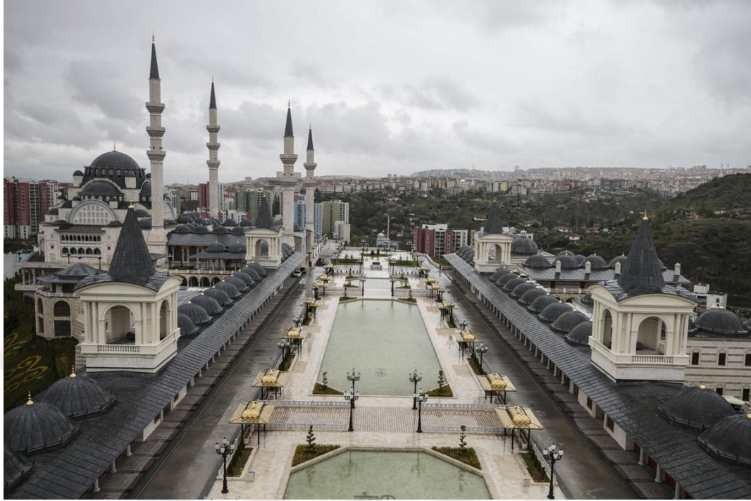
Figure 4.10 General View of The Great Ankara Mosque (source: AA, 2019)
