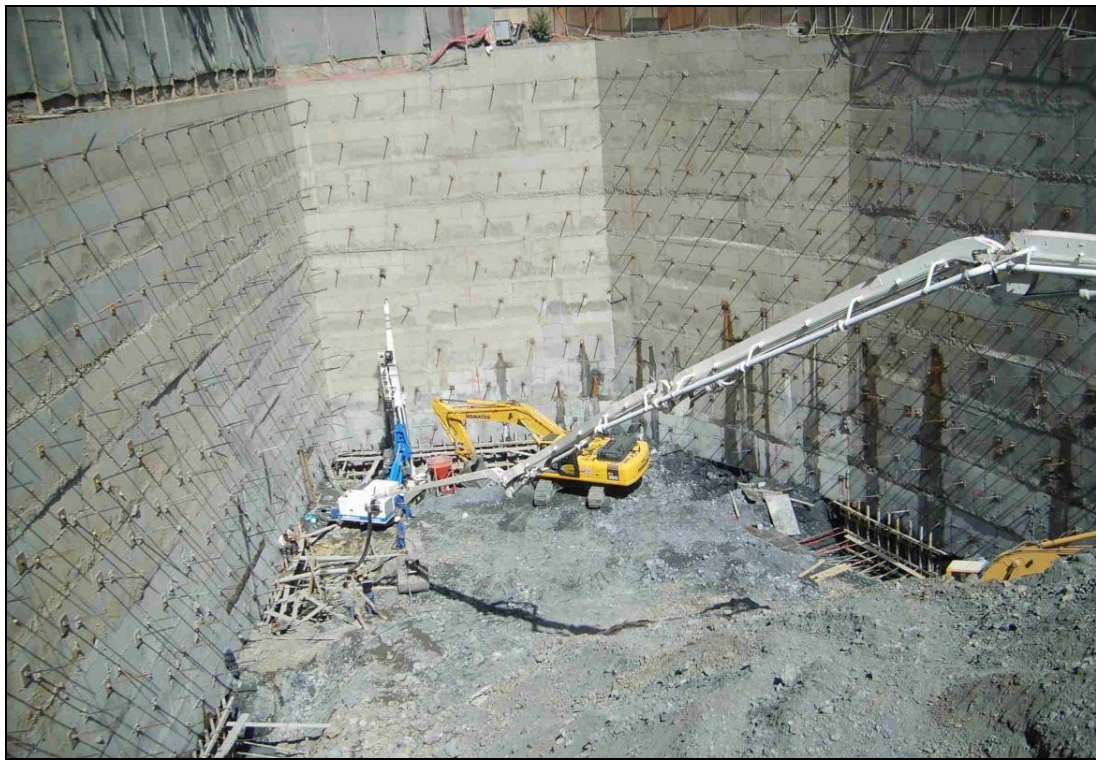
Figure 3.24 Construction of the last stage walls at the Part-1.
