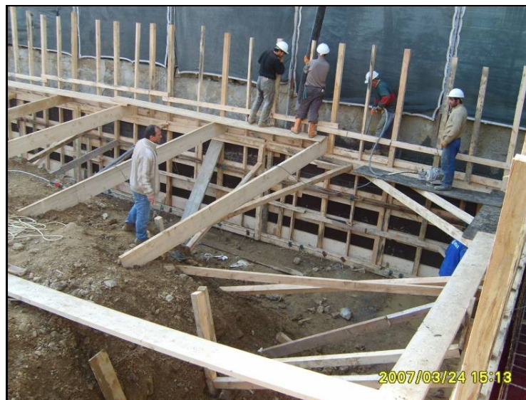
Figure 3.10 Formwork support installation.
