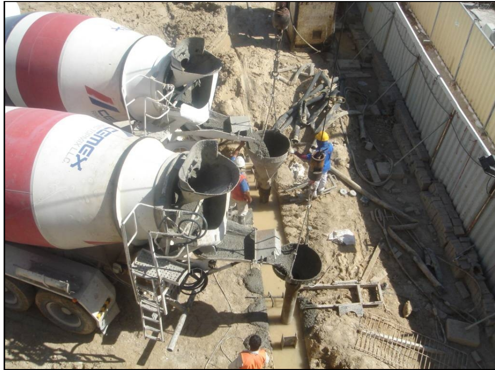
Figure 2.28. Concreting in progress.
