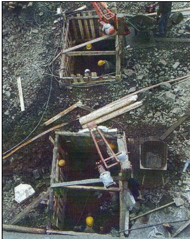
Figure 2.16 Construction of the primary panels.
