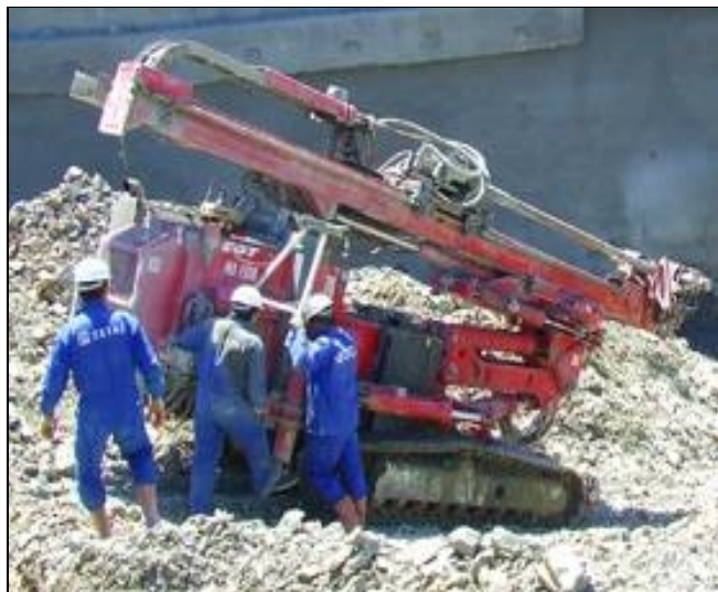
Figure 2.10 Track mounted drilling rig, EGT MD 1500.
