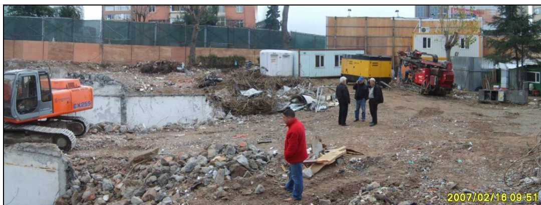
Figure 3.5 General site condition and site preparation works.
