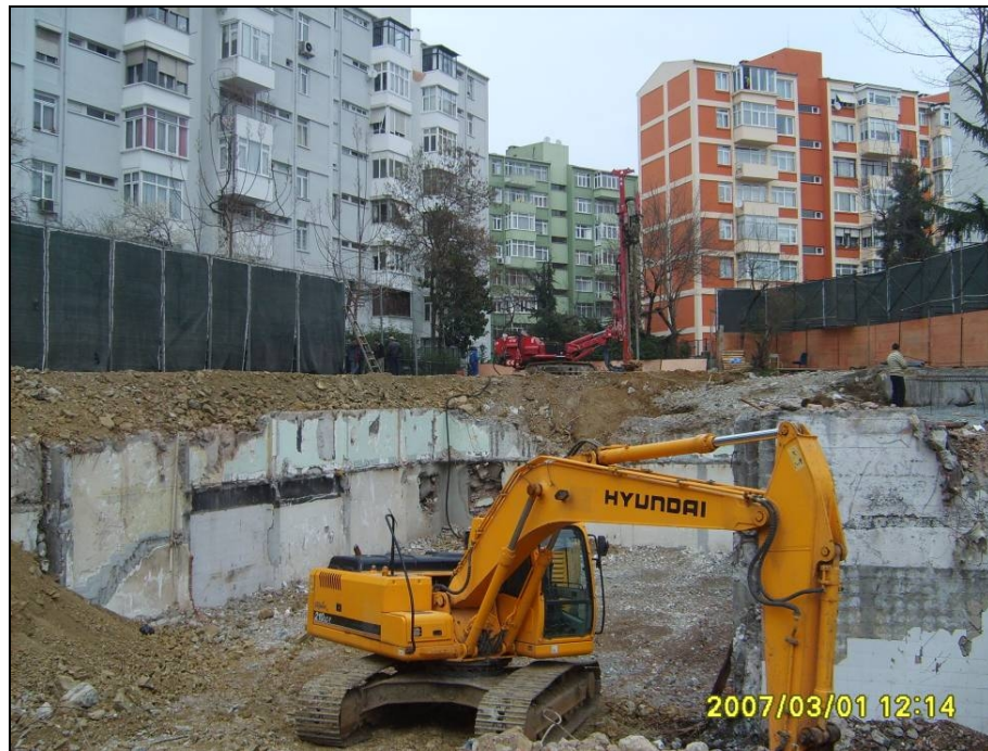
Figure 3.6 Demolition and site preparation works going on concurrently with micro pile construction.
