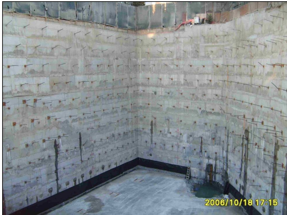
Figure 3.25 Part-1 just after the retaining walls were completed.
