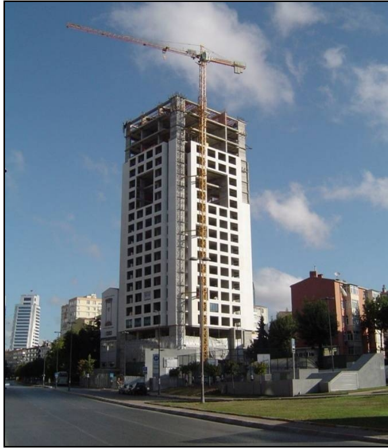
Figure 3.2 Point Hotel Barbaros, during the construction, July 2008.
