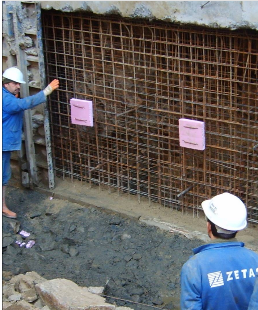
Figure 2.31. Placing of wire mesh reinforcement of the panel and placing of the styrofoam blocks for the anchor head installation (Zetas, 2007).
