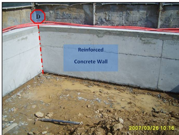
Figure 3.11 First stage reinforced concrete wall.
