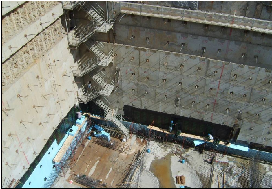
Figure 2.1 Anchored cast in-situ reinforced concrete retaining wall construction (Zetas Zemin Tenolojisi A.S., 2008).
