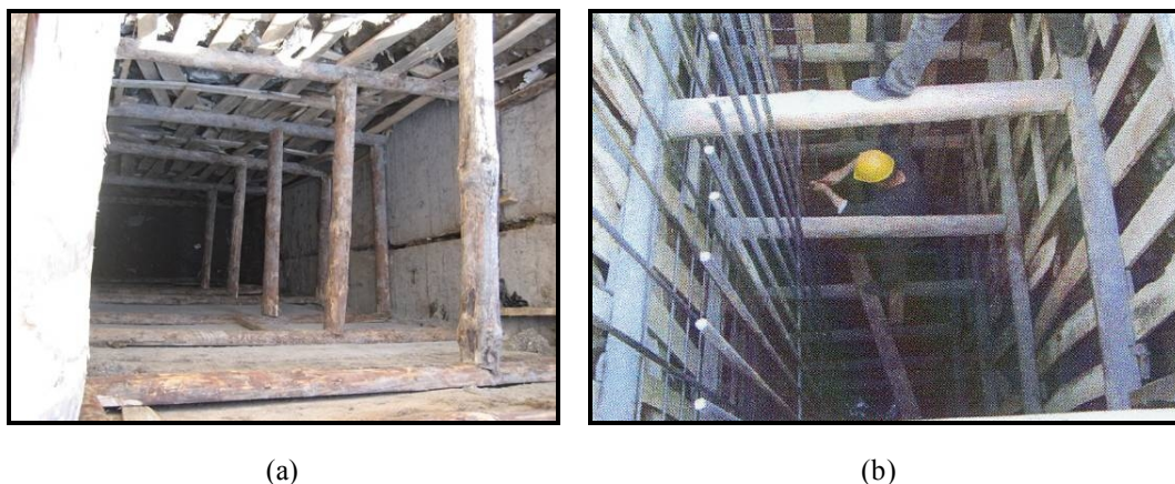
Figure 2.17 A typical manual caisson support configuration. (a) Excavation, (b) Placing of reinforcement.
