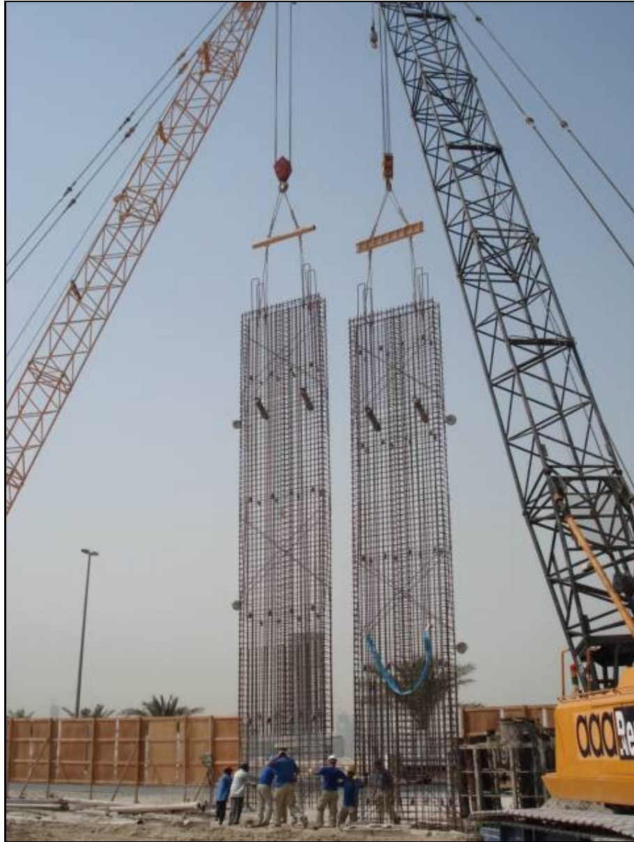
Figure 2.26 Reinforcement placing.
