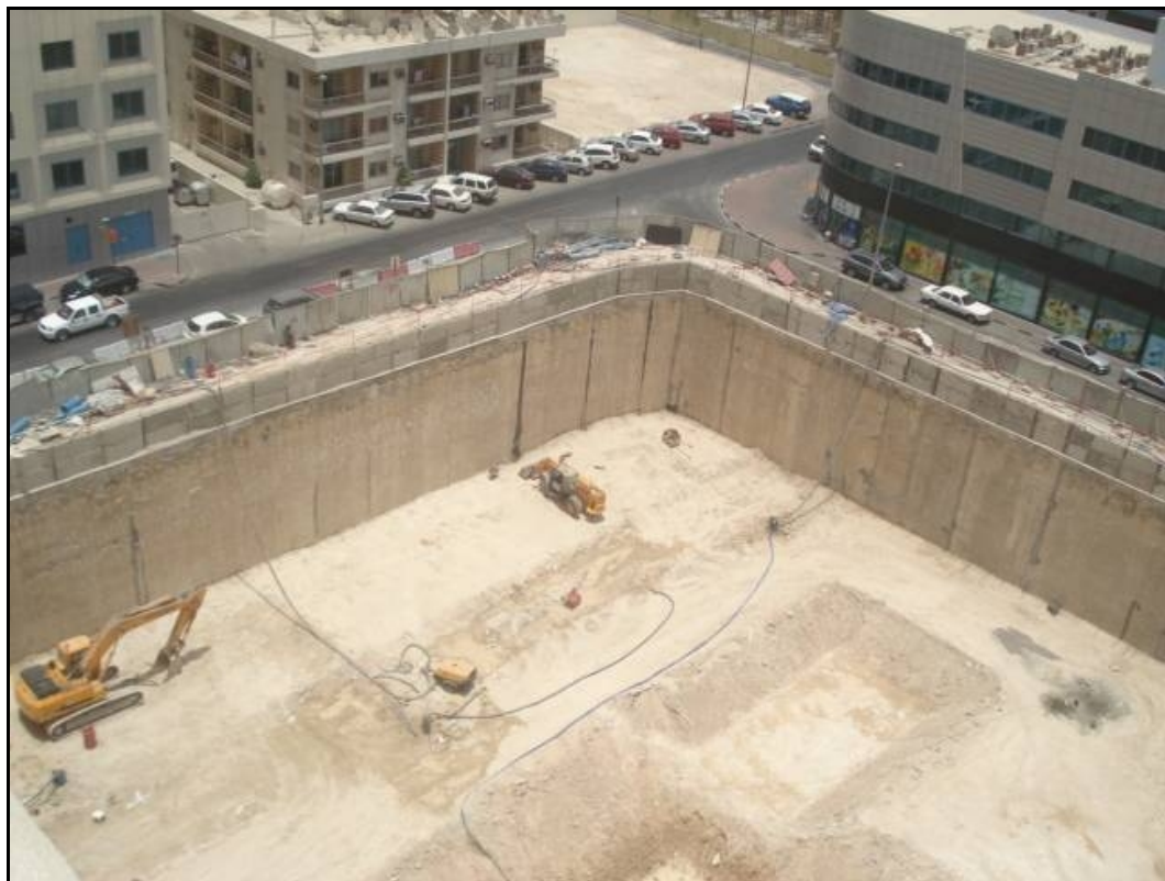
Figure 2.19 Deep excavation with diaphragm wall in the city center of Dubai (Zetas, 2007)
