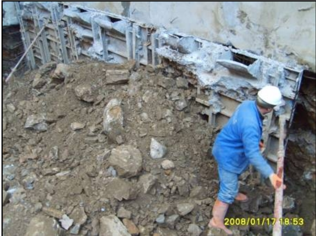
Figure 2.32 Placing of single sided metal frame formwork panel with back fill method (Zetas, 2007).
