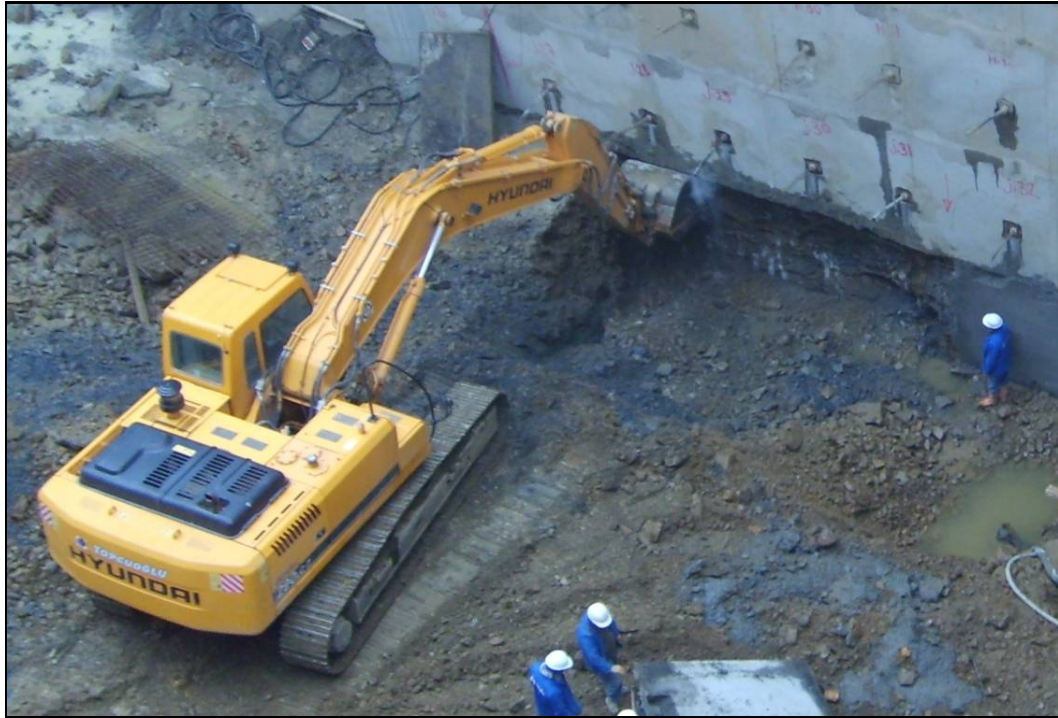
Figure 2.30. Excavation of the RC wall segment (with pre-stressed ground anchors) at the later stage of the construction (Zetas, 2007).
