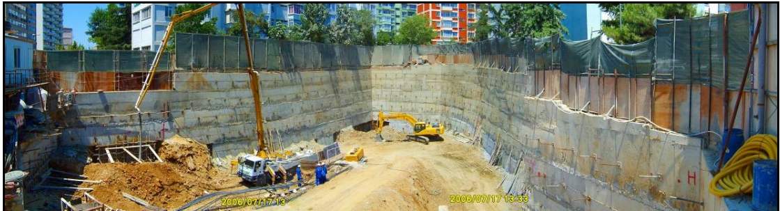
Figure 3.14 Retaining wall construction progress on the 17 th day of July.
