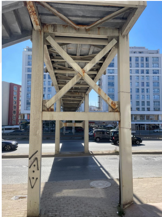
Figure A.2: Support End Column
