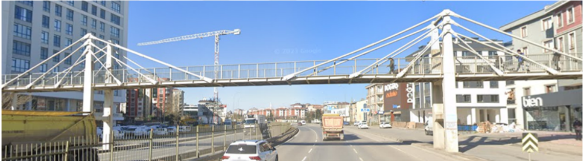
Figure 3.1: Front View of the Taşdelen Cable-Stayed Pedestrian Bridge
