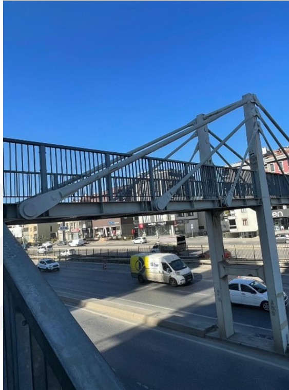
Figure 4.6: Tension cables on the bridge
