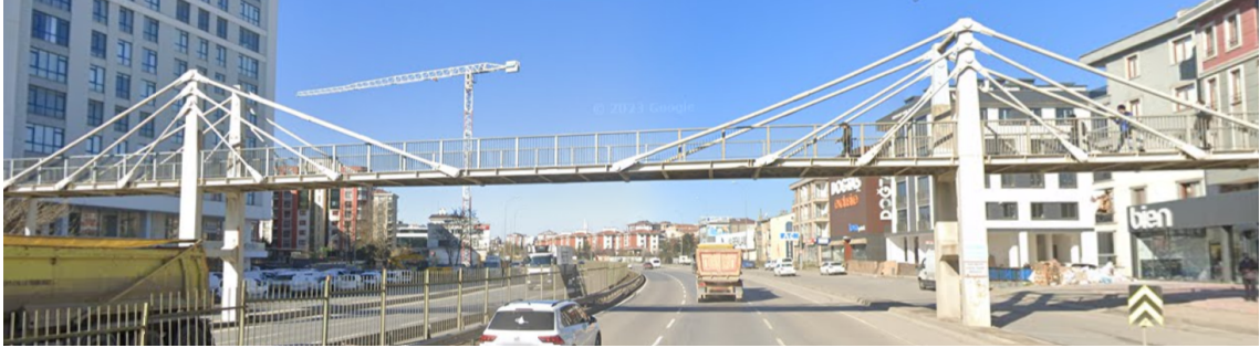
Figure A.1: Tasdelen Cable-Stayed Pedestrian Bridge
