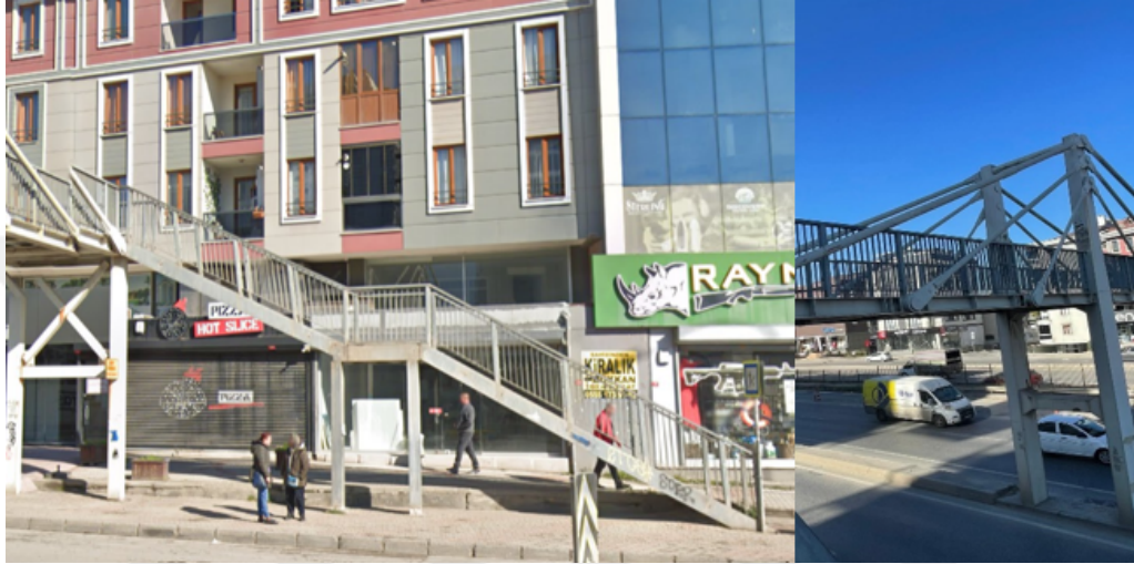
Figure 4.4: Support columns, stair columns and pylons
