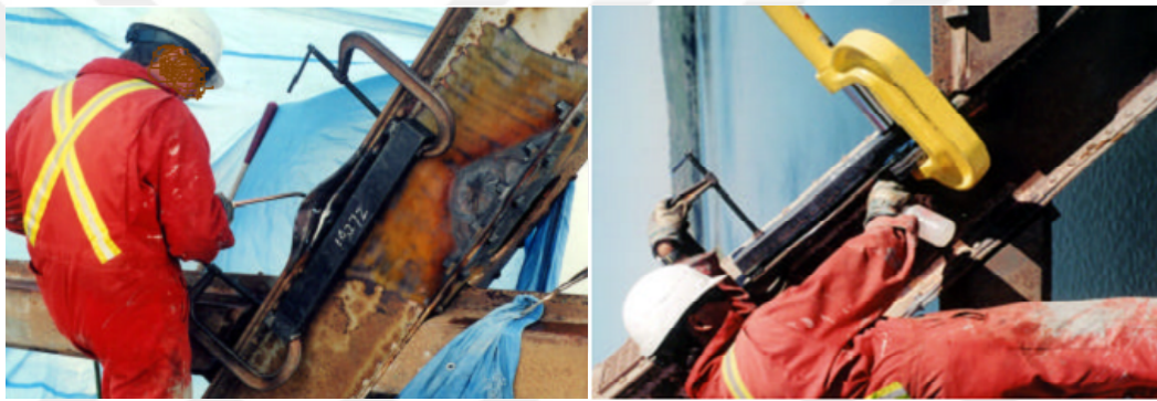
Figure 2.3. Heat treatment of steel girders [7].
