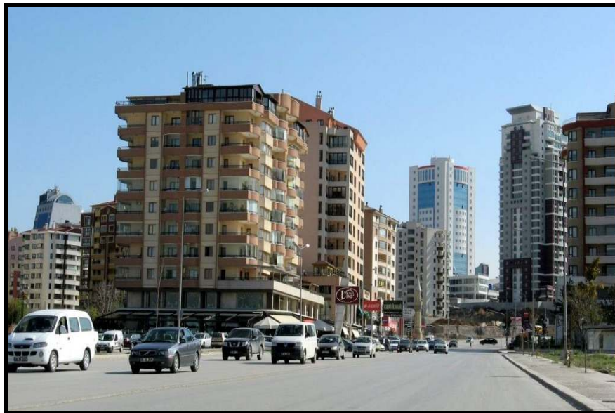
Figure 4.12. A new picture of 48. Road
