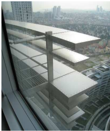
Figure 4.10: Shading devices from inside.
