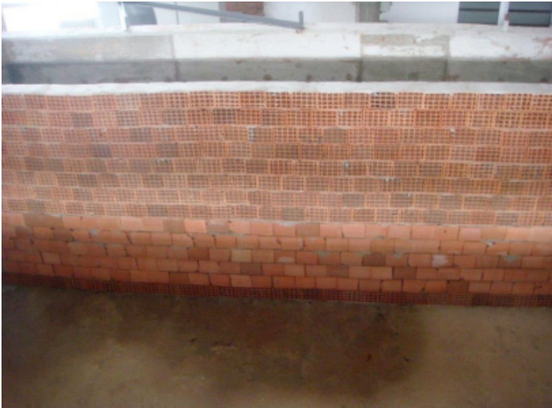
Figure 4.5: Buffle Blocks at the entrance of the reservoir
