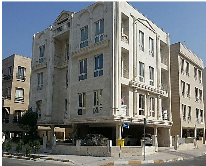
Figure 4.15: Case Study External View (Source: Author)
