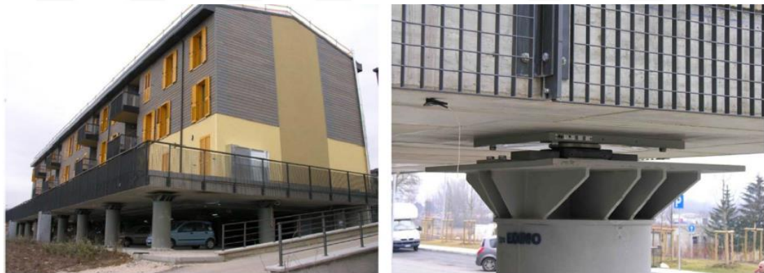
Figure 2.14 The implementation of BIS [71]
