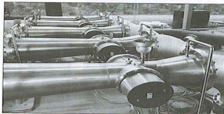
Figure 1.7 Typical Closed-channel UV System and its Typical Installations (Metcalf&Eddy, 2003).
