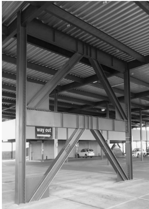
Figure 1.4: Eccentrically braced frames in practice ( www.civilweb.ir )
