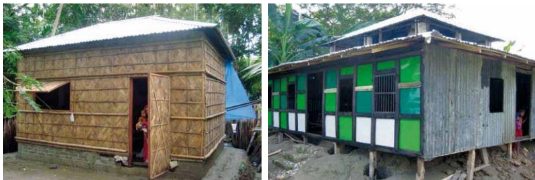
Figure 2.3 Core shelter of Bangladesh and its upgrading (UN-HABITAT and IFRC, 2010)
