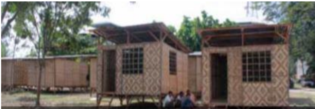
Figure 2.6 Shelter example from Philippines (do Nascimento, 2015)
