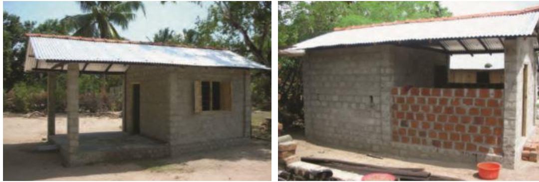
Figure 2.8 Complete core shelter in Sri Lanka and its durable upgrade (Ashmore, 2008)
