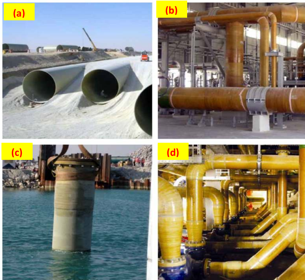
Figure 3.9 (a) GFRP pipes underground application (O&G and Wastewater application); (b) GFRP industrial application; (c) GFRP underwater application (Bridge, O&G platforms..); (d) GFRP marine application (vessels, submarine...) [23].
