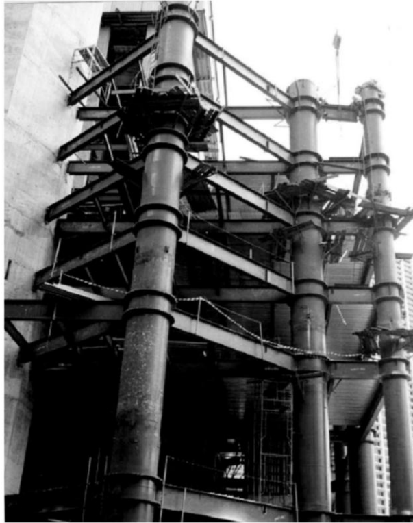
Figure 2.23 Circular steel tubes before pouring concrete (Liew and Xiong, 2012)
