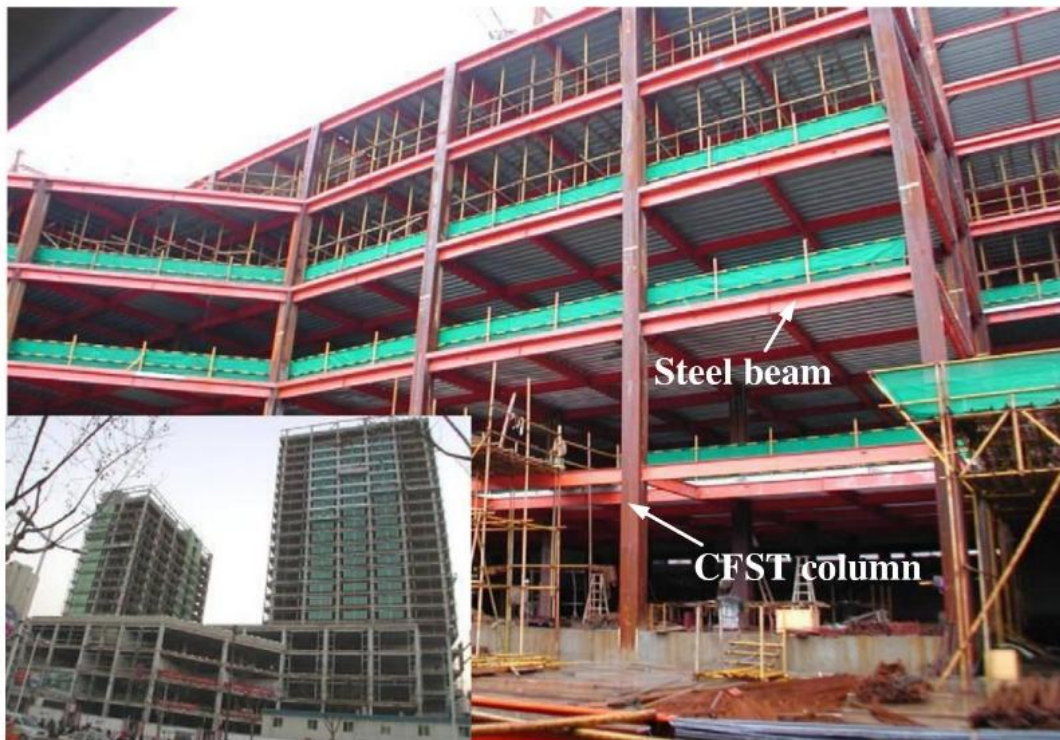
Figure 2.24 Ruifeng building, China, 2001 (Han et al. , 2014)
