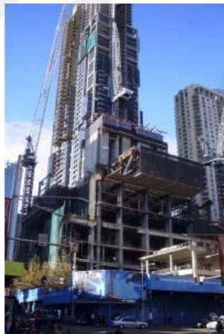
Figure 2.6 Latitude, a building in Sydney, Australia (Tao et al., 2008b)
