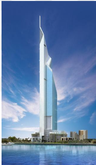
Figure 2.8 Dubai tower in Doha (Davids et al., 2008)
