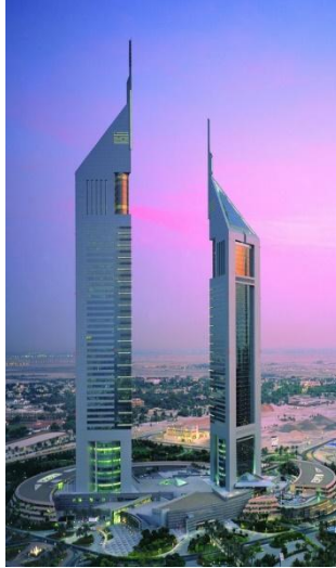
Figure 2.7 Emirates Towers in Dubai (Davids et al., 2008)
