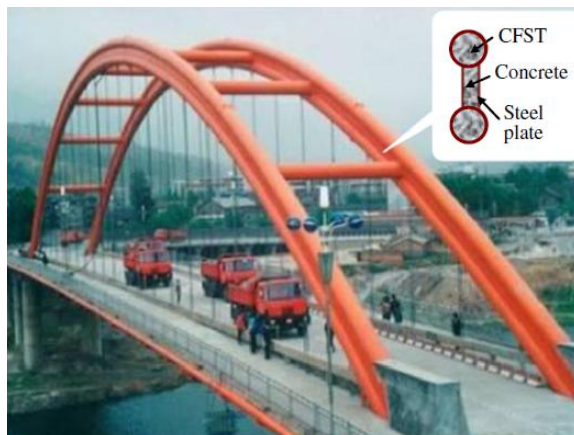
Figure 2.12 Wangcang East River CFST arch bridge (Han et al., 2014)
