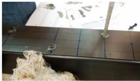
(d) Application of epoxy and installation of bolts through holes
