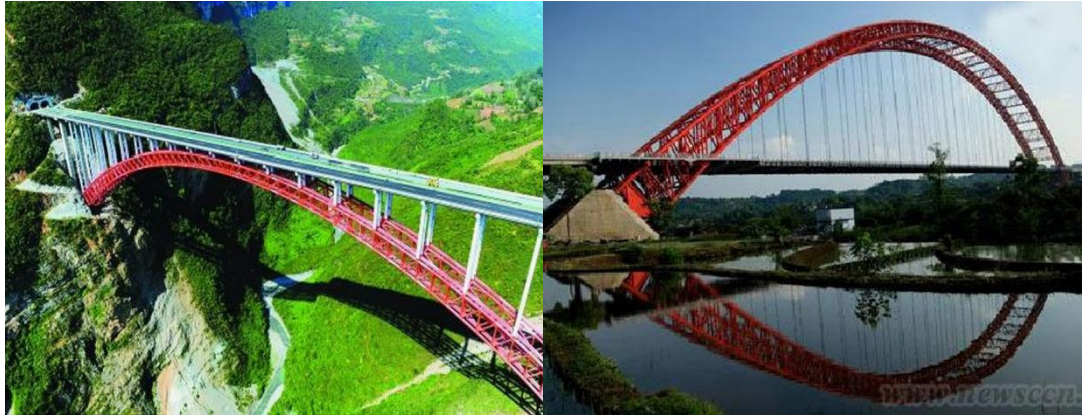
(a) Zhijing Bridge
