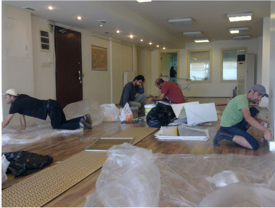
Figure 6.4. çapul.tv office section during the time of renovation
