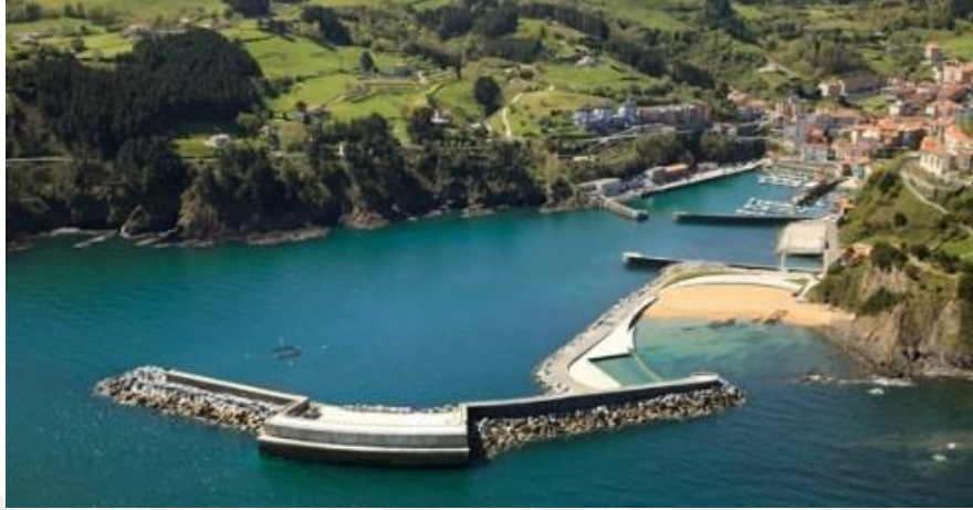
Figure 2.6. Mutriku breakwater OWC
