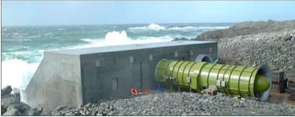
Figure 2.3. LIMPET OWC plant
