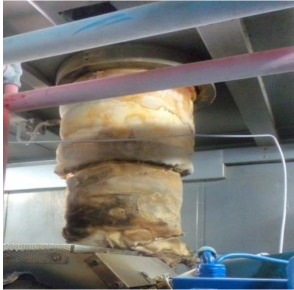
Figure 3.7 Exhaust Filter
