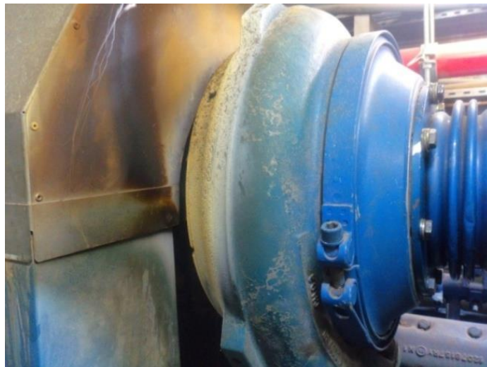
Figure 3.4 Turbocharger
