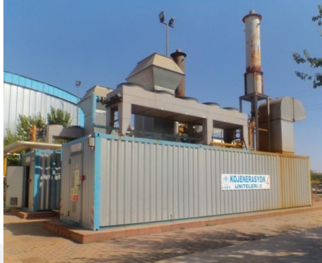
Figure 3.1 Biogas Engine Powered Cogeneration Sytem
