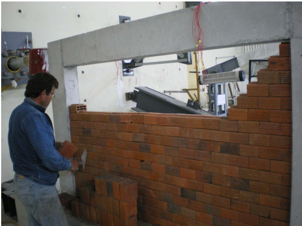
Figure 3.8 Locked brick usage during construction
