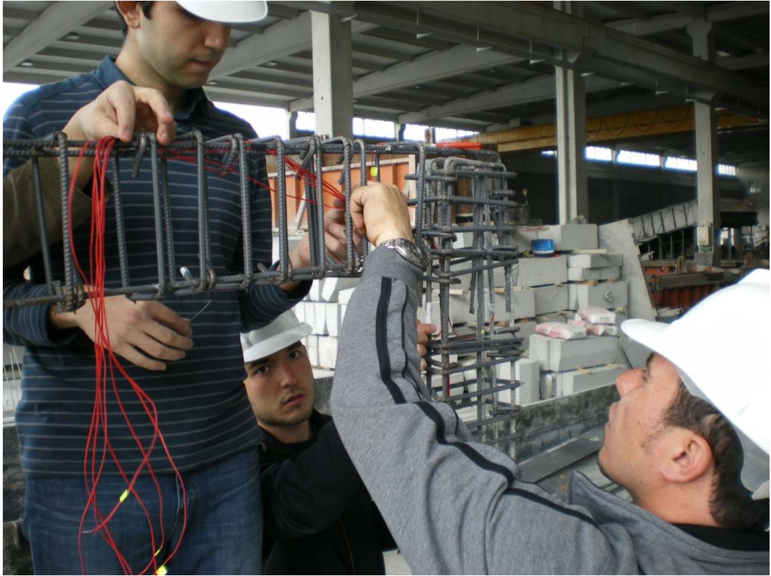
Figure 3.22 Forming of connecting cables
