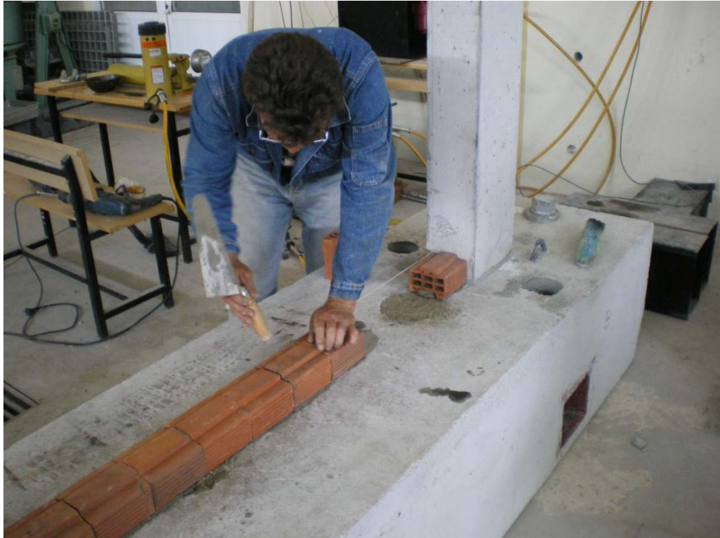
Figure 3.7 First row of locked bricks
