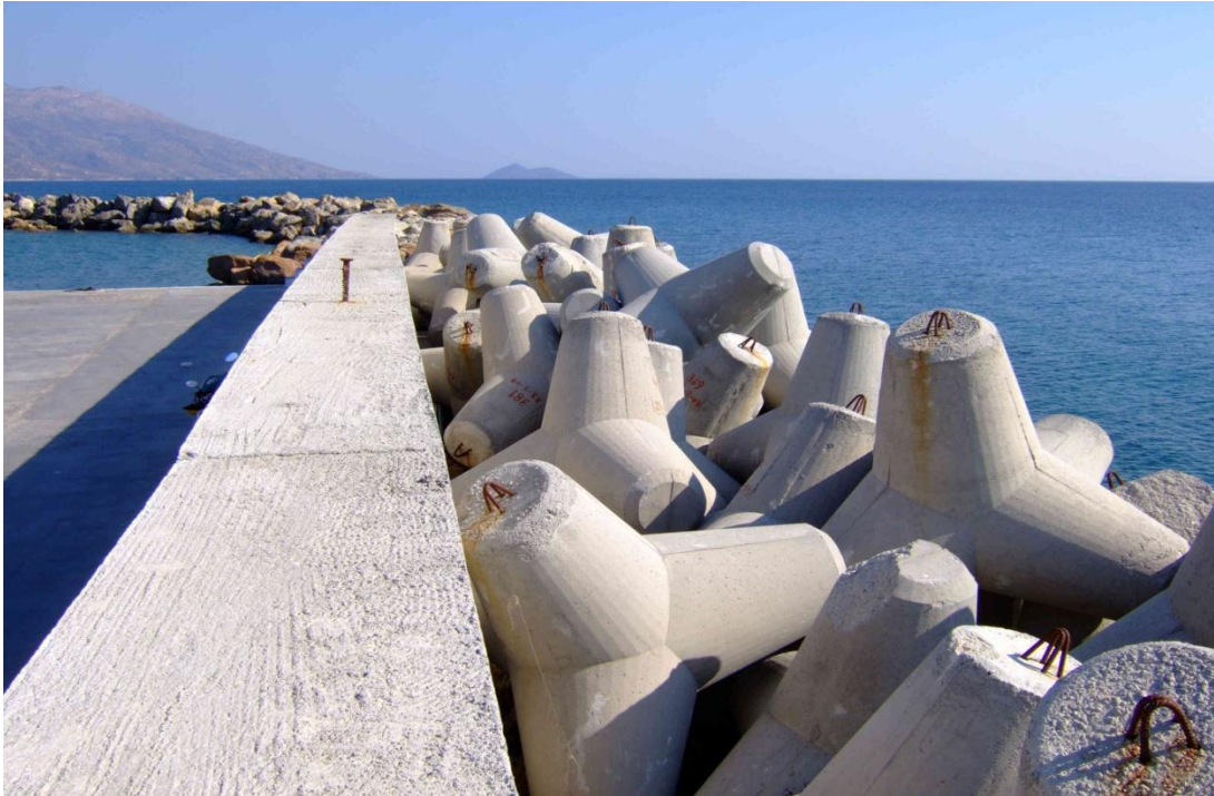
Figure 3.4 : Tetrapods breakwater, Japan (URL-7)
