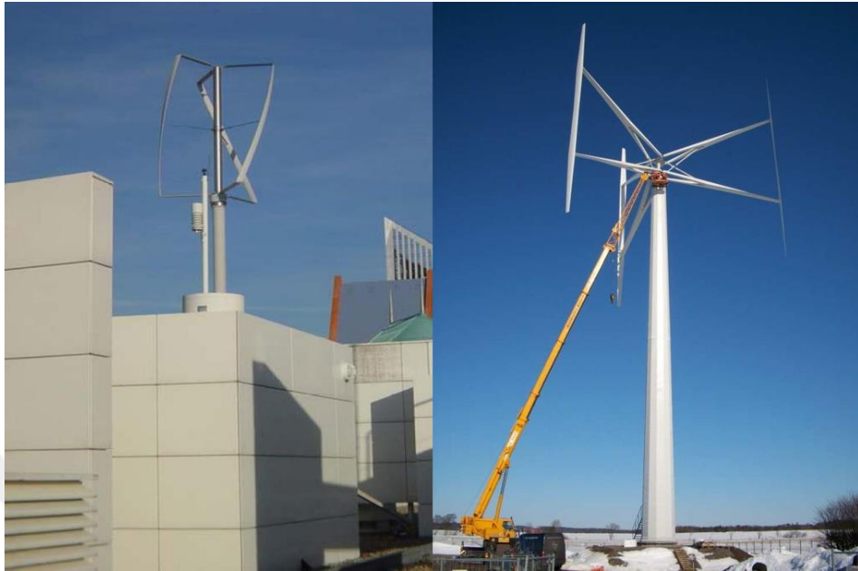
Figure 1.3 Three bladed helical Darrieus type VAWT(left); three bladed H-rotor Darrieus type VAWT (right) (Ragheb,2015; D'Ambrosio & Medaglia, 2010)
