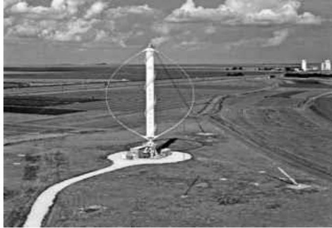
Figure 1.4 34 m Darrieus type vertical axis wind turbine located and tested in Sandia Labs.in Texas U.S. (Sandia, 2015)
