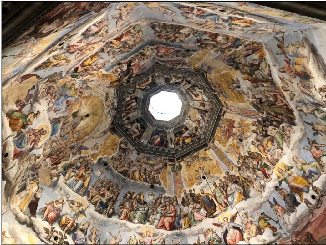
Figure 3.17 . Dome of Cathedral of Santa Maria de Fiore from interior [50].
