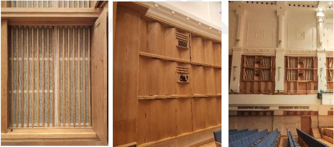
Figure 33. Retracted, half-retracted and closed states of the variable absorption system in Bilkent Music Hall, respectively (photos by the authors)
