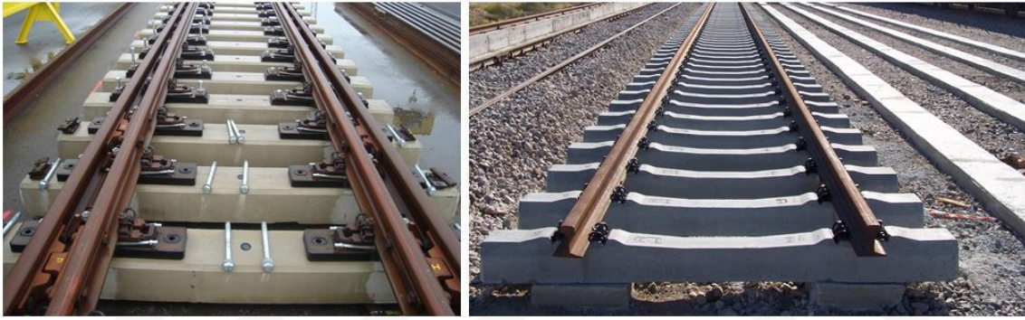
Resim 4.5 Mono blok beton travers (TCDD 2018).
