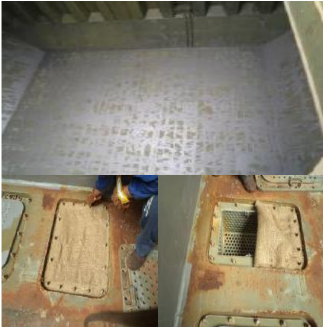
Figure 2.5 : General view of ship's hold (upper) and hold bilges (bottom left&right).
