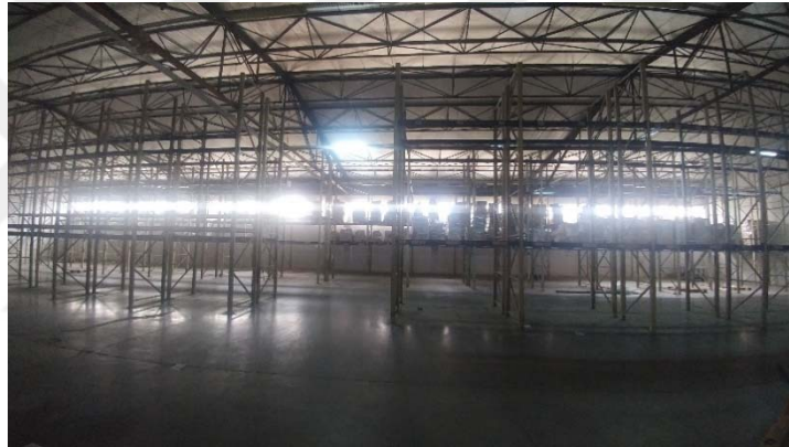
Figure 5.10 Front view from the depot (Personal archive, 2018)
