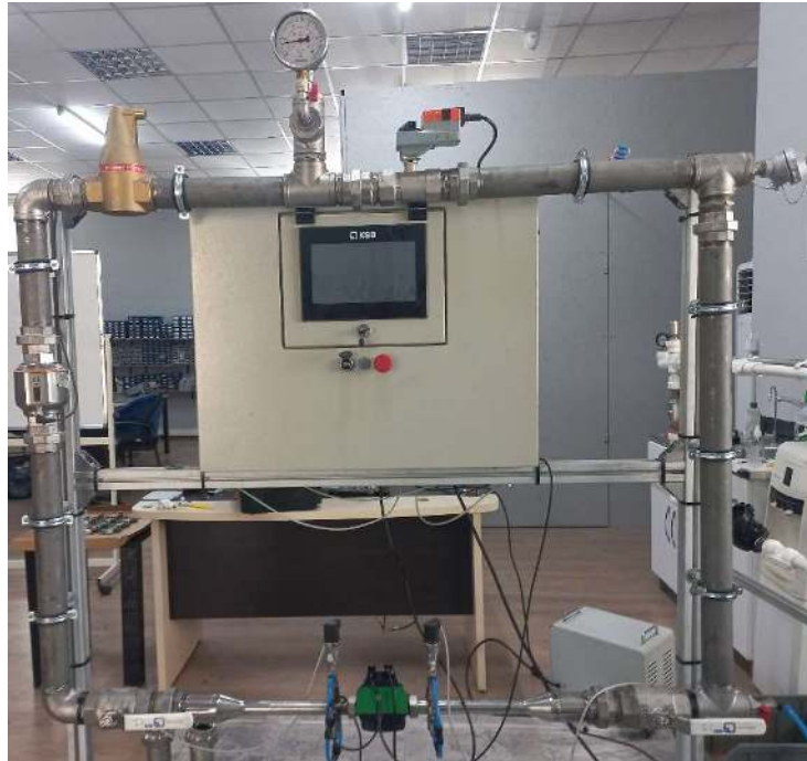
Figure 13: Photograph of the experimental test rig.
