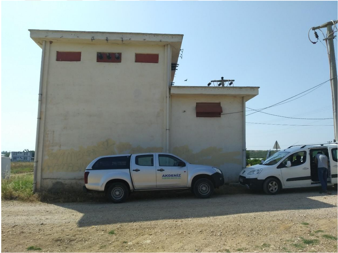
Figure 4.1 Distribution Station of AKDENİZ EDAS
