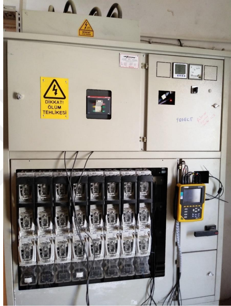
Figure 4.3 Main Distribution Panel of AKDENİZ EDAS DS
