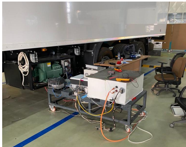
Figure 3.17. Stages Of The Energy Storage System-2.
