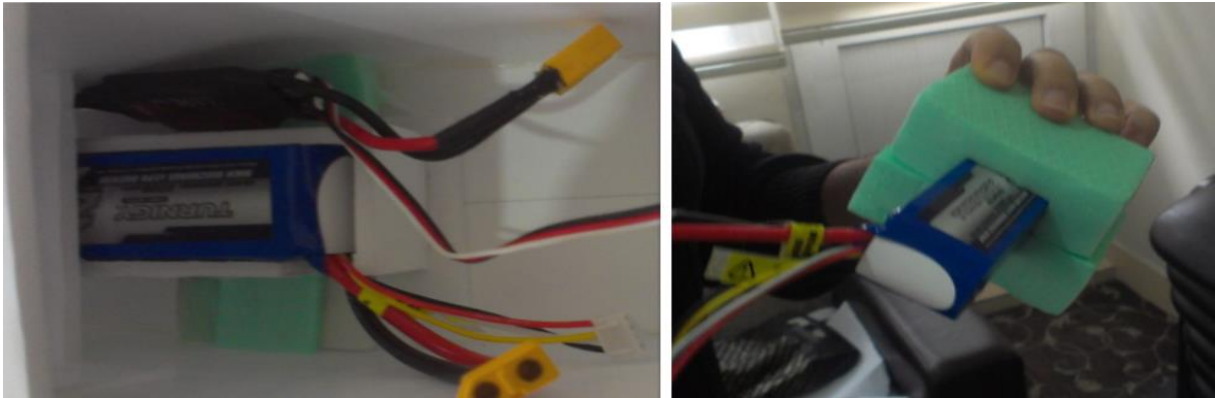
Fig. 6.8 Installation of power system
