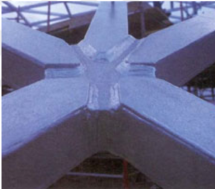
Figure 3.57 End-Face Connector WABI-1 (Stephan et al., 2004)
