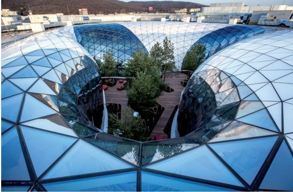
Figure 4.11 “Tornado” facade from outside (Metal Yapi)
