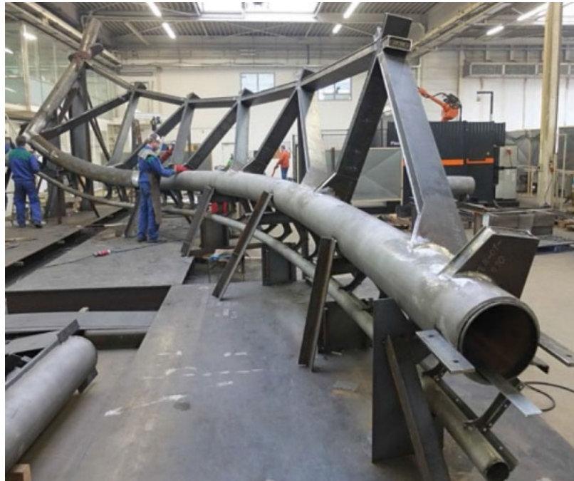
Figure 3.42 Fabrication of edge beam (Seele Pilsen)
