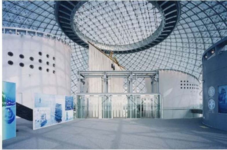
Figure 3.22 South Pole Dome interior view, Antarctica (Andrieu, 2000)
