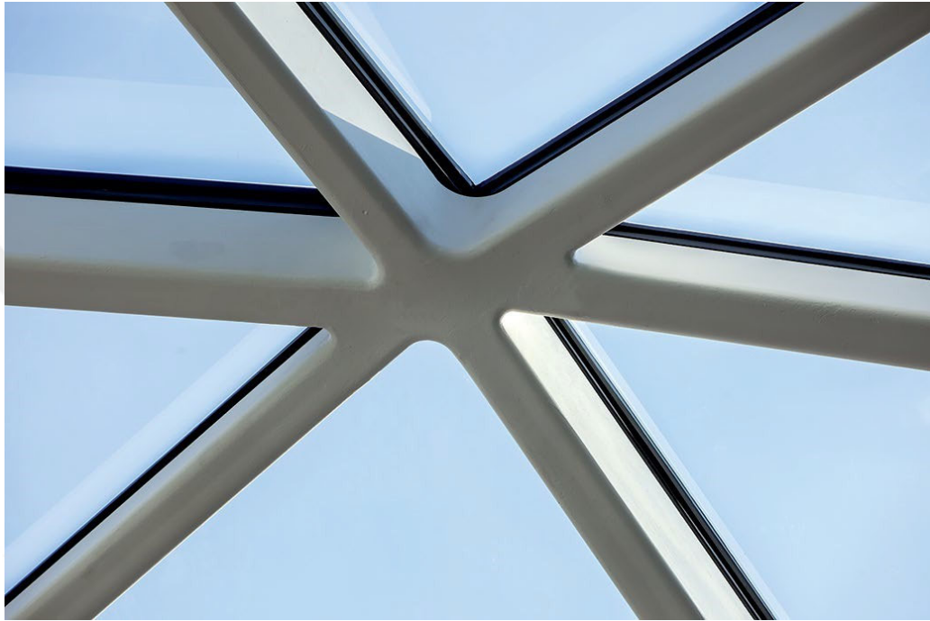
Figure 4.15 Finished node installed on site (Metal Yapı)
