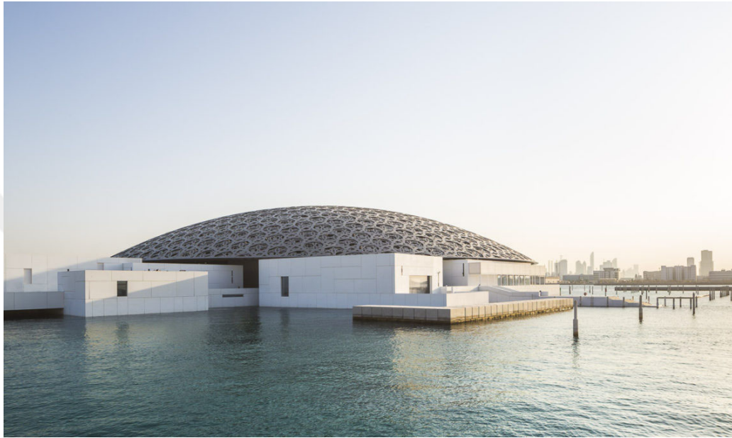
Figure 3.34 Abu Dhabi Louvre, UAE (Halbe, 2017)
