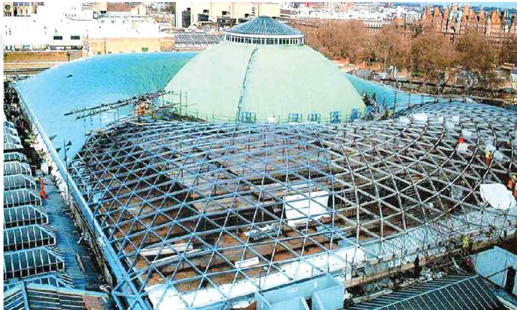
Figure 3.51 British Museum Great Court Roof, glass installation (Waagner Biro)
