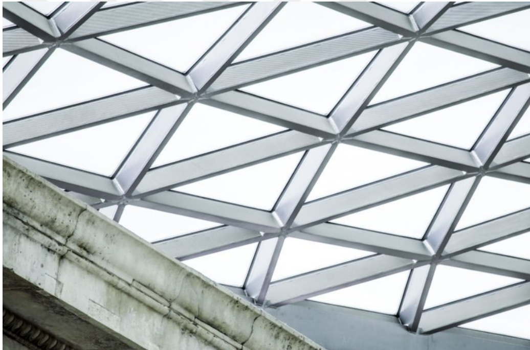
Figure 4.8 Node with welds (Waagner Biro)
