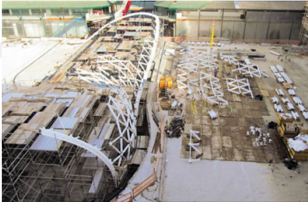
Figure 3.45 Erection of the canopy on site (Seele-Austria)
