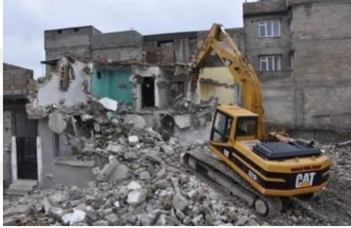
Figure 2.4. Demolition in Şahinbey Municipality
