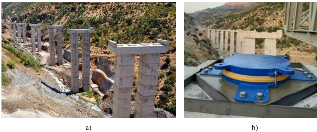
Figure 2.5. View from the construction site of Bitlis Viaduct (a), and installation of a friction pendulum on top of the pier (b)
