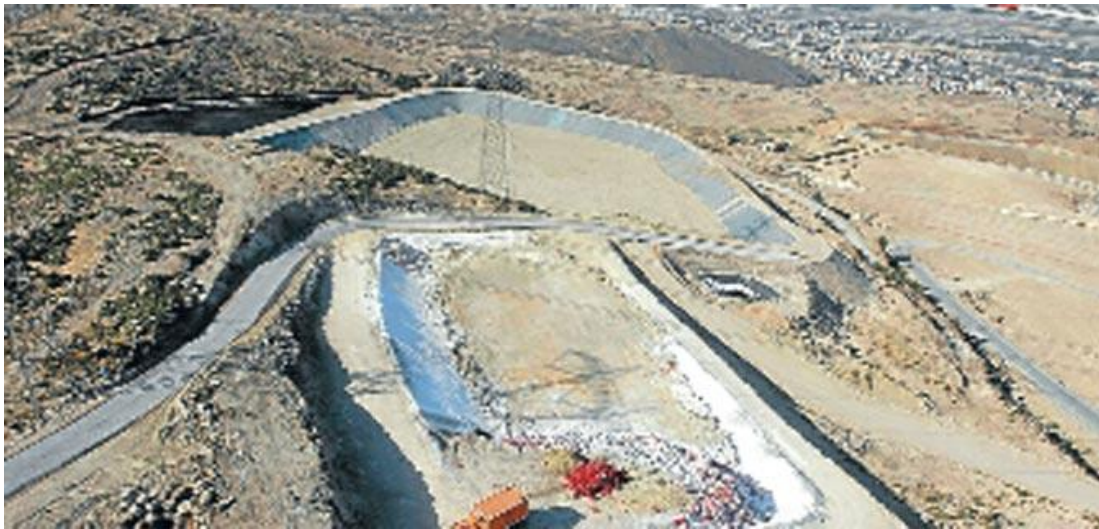
Fig 4.1 Harmandalı New Lot Construction
