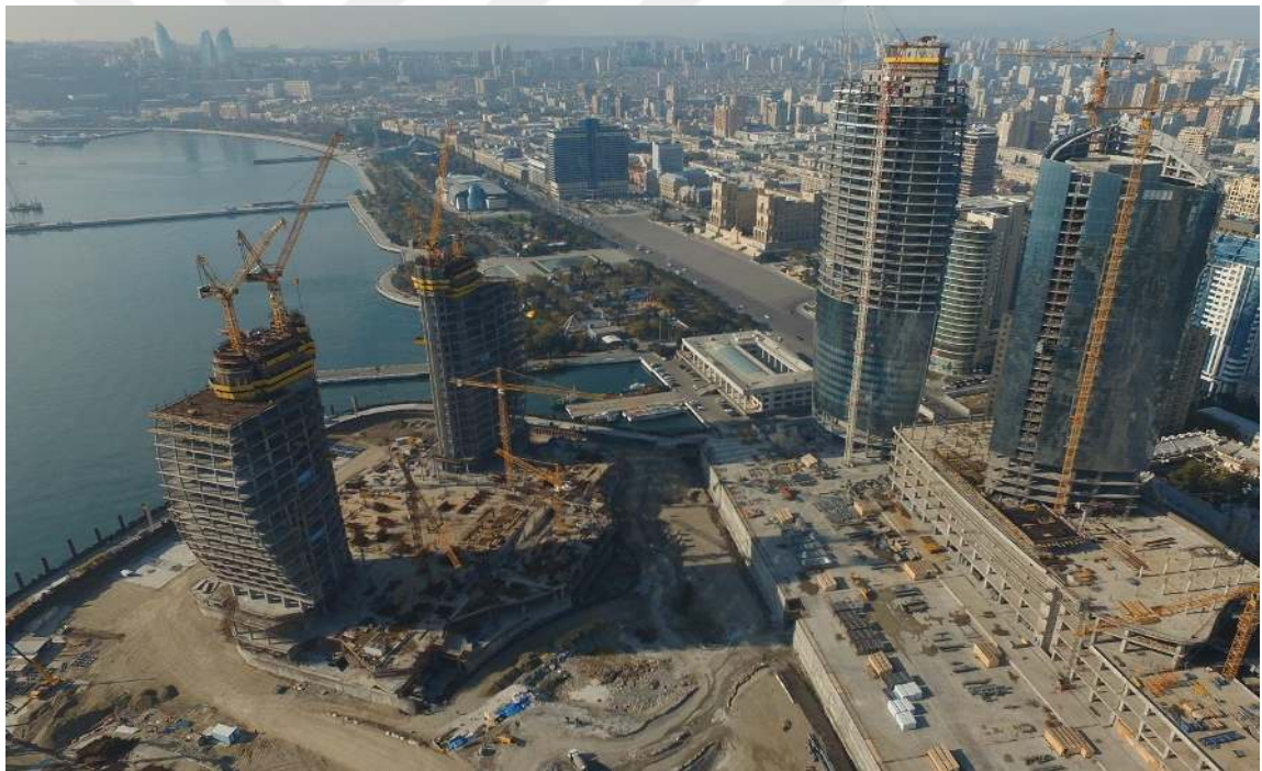
Figure 5: ILK construction Port Baku Residence project
