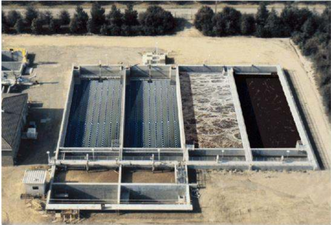
Figure 2.2 A general view of SBR type WWTP
