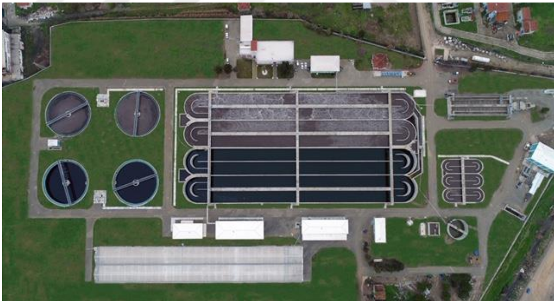
Figure 2.1 A general view of WWTP
