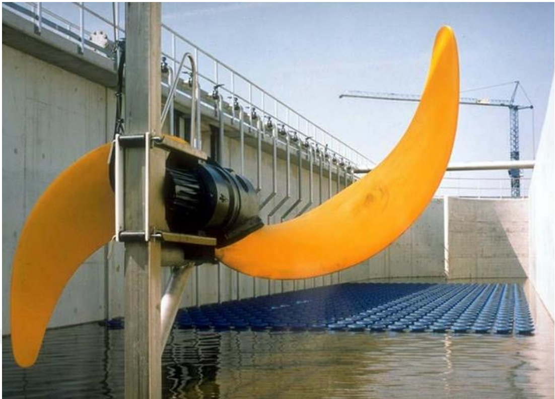
Figure 2.10 A general view of oxidation ditch
