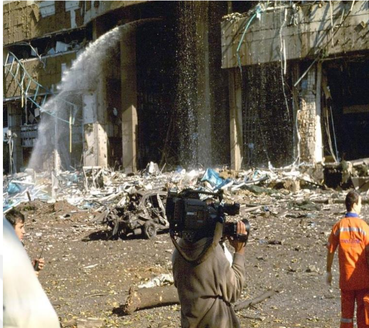
Image 7. On the Day of HSBC Explosion, November 20 th , 2003. This figure shows the damage to the HSBC building inflicted by the explosion. (Photo: Reyhan Erkenci).
