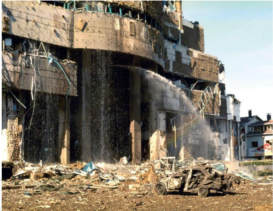
Image 13. On the Day of HSBC Explosion, November 20 th , 2003. This figure shows the damaged HSBC building after the terrorist attack in Levent. (Photo: Reyhan Erkenci).
