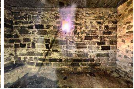
c) Z07 oda güney cephe
