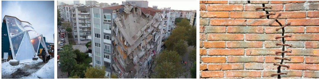
Figure 2.32. (1) Building Raincoat prototype for smart city in Toronto by Sidewalk Labs (retrieved from on 23.11.2020), (2) Demolished building after İzmir Earthquake in 2020 (retrieved from https://www.aa.com.tr/ on 23.11.2020), (3) Cracks in Plaster/Masonry Walls (retrieved from https://www.civilax.com/ on 23.11.2020)
