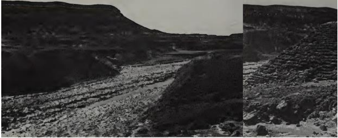
Figure 1.2. The Ruins of Sadd el-Kafara Dam (Smith, 1972)
