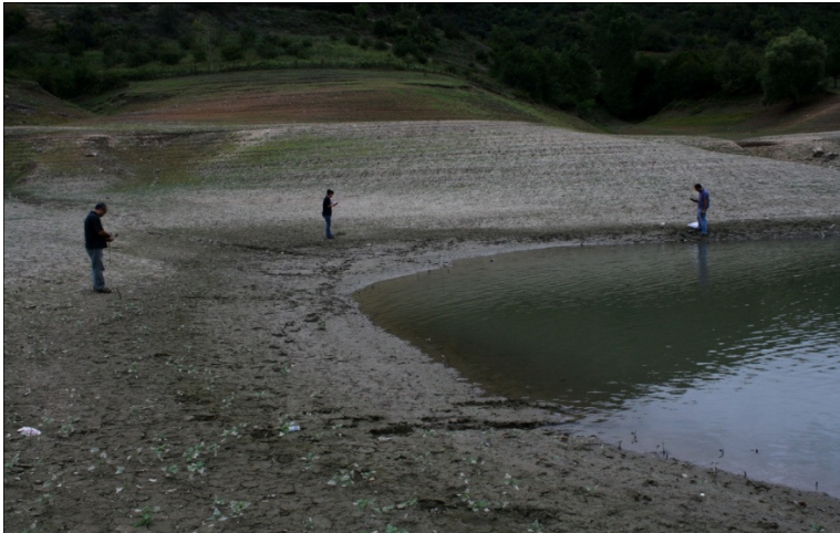
Photo 2. Station 17. Hasanlar Dam in Düzce.
